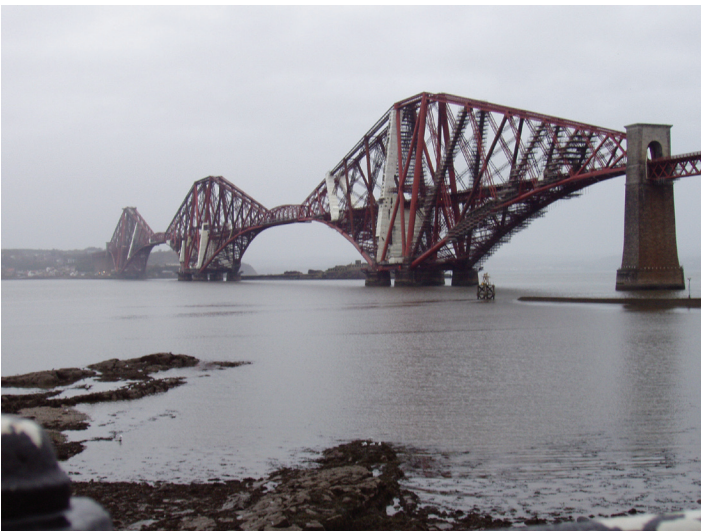
The Forth Rail Bridge (1883-90), near Edinburgh
