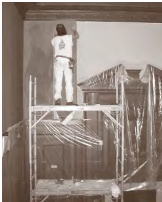
Restoring grandeur: hanging historic wallpaper in the Millikin room restoration, 2000.
