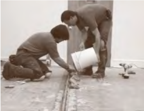
Laying rails for compact storage in the Peterson Room, 2002.
