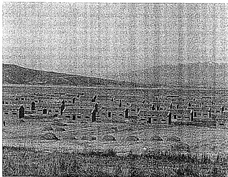
Photo 12.1 Longzang resettlement village in Ningxiu, Zeku County (Photograph © Jarmila Ptackova, July 2008)
