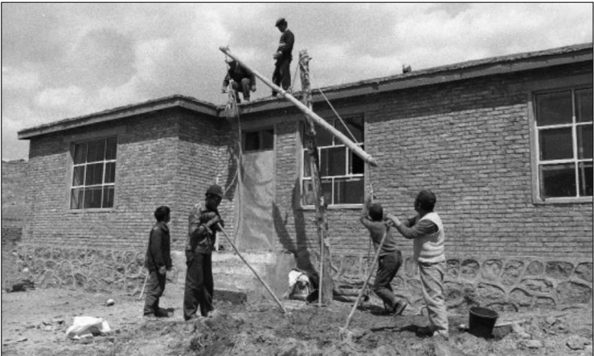
**Figure 5:** *Each House had New Double-paned Windows. Here Residents are Supplementing the Existing Roof*
