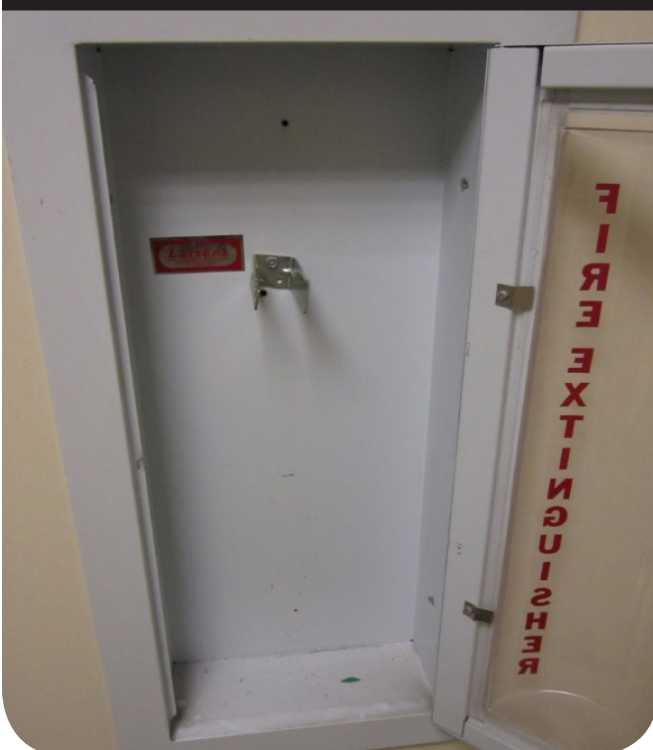
Missing Extinguisher
