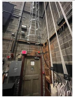
Fixed ladders are permanently attached to structures or equipment. They often provide access to catwalks, grids and loading bridges. When used in performance either as a scenic element or as access from trap door pits, they must conform to the same standards.
