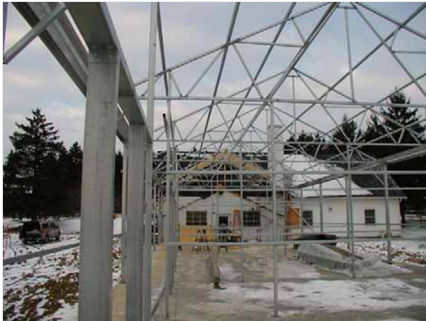
Hallway and rooms separations
