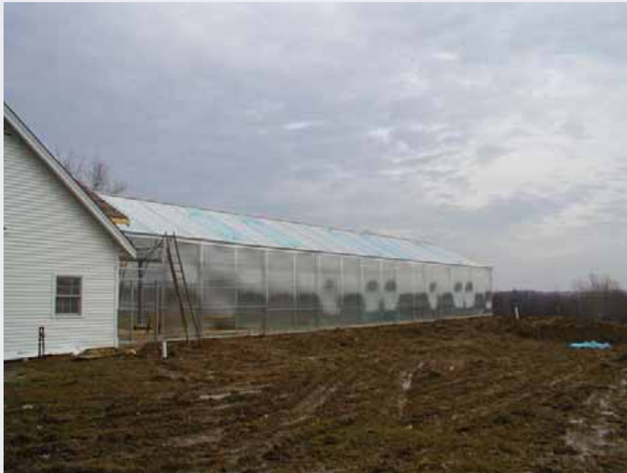
Outdoor poly walls installation is finished
