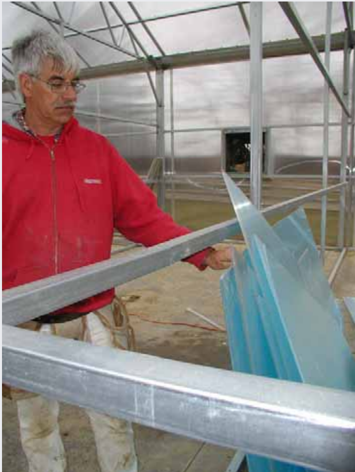
8 mm double poly walls coated for condensation resistance and UV protection
