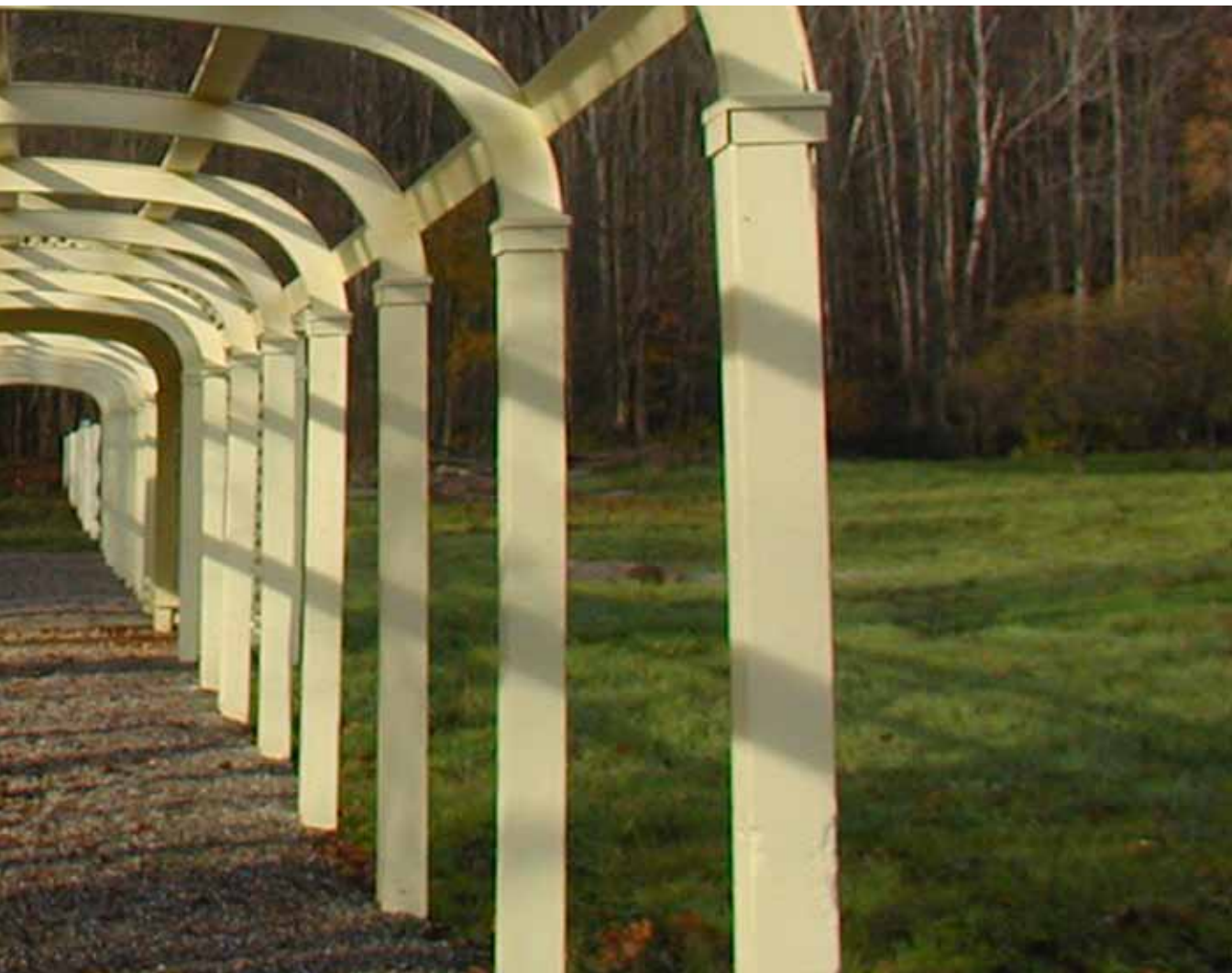
Wade gardens Grape Arbor restoration project at Valley Ridge Farm
