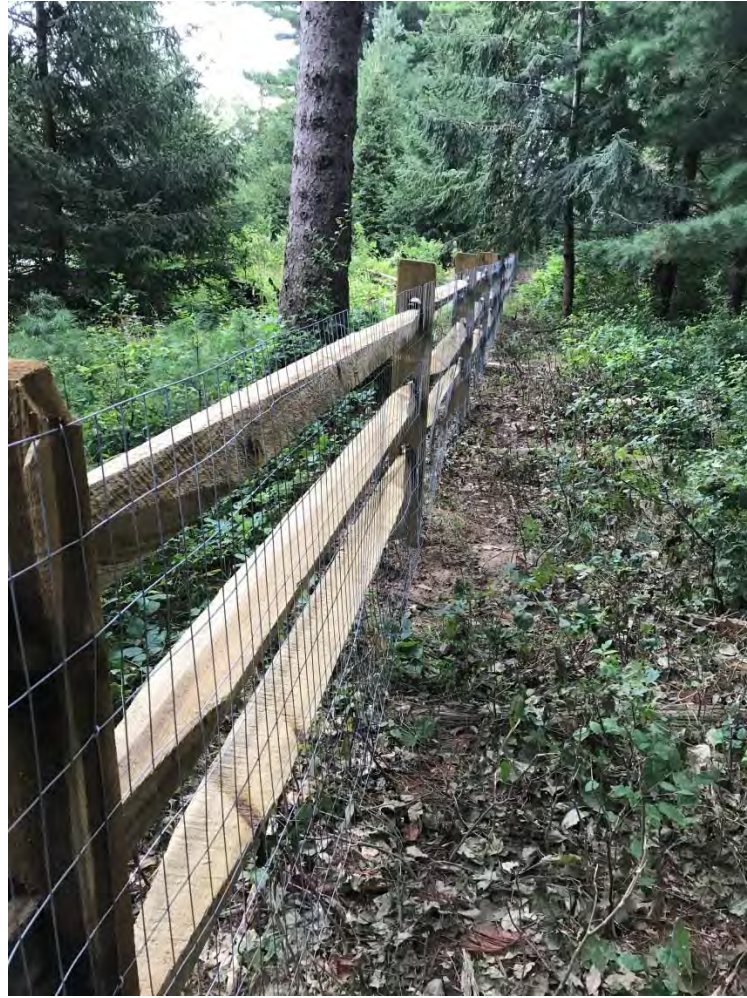
Split rail fencing was installed along Cedar Road property lines.
