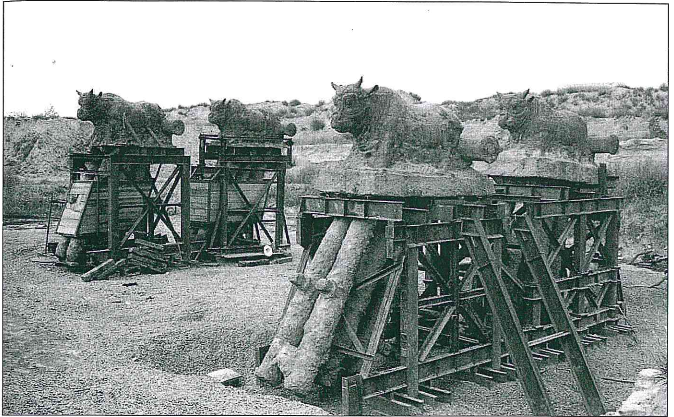
Figure 6: These four cast-iron oxen of the eastern anchorage, with their six raked support pillars, were recently excavated.
