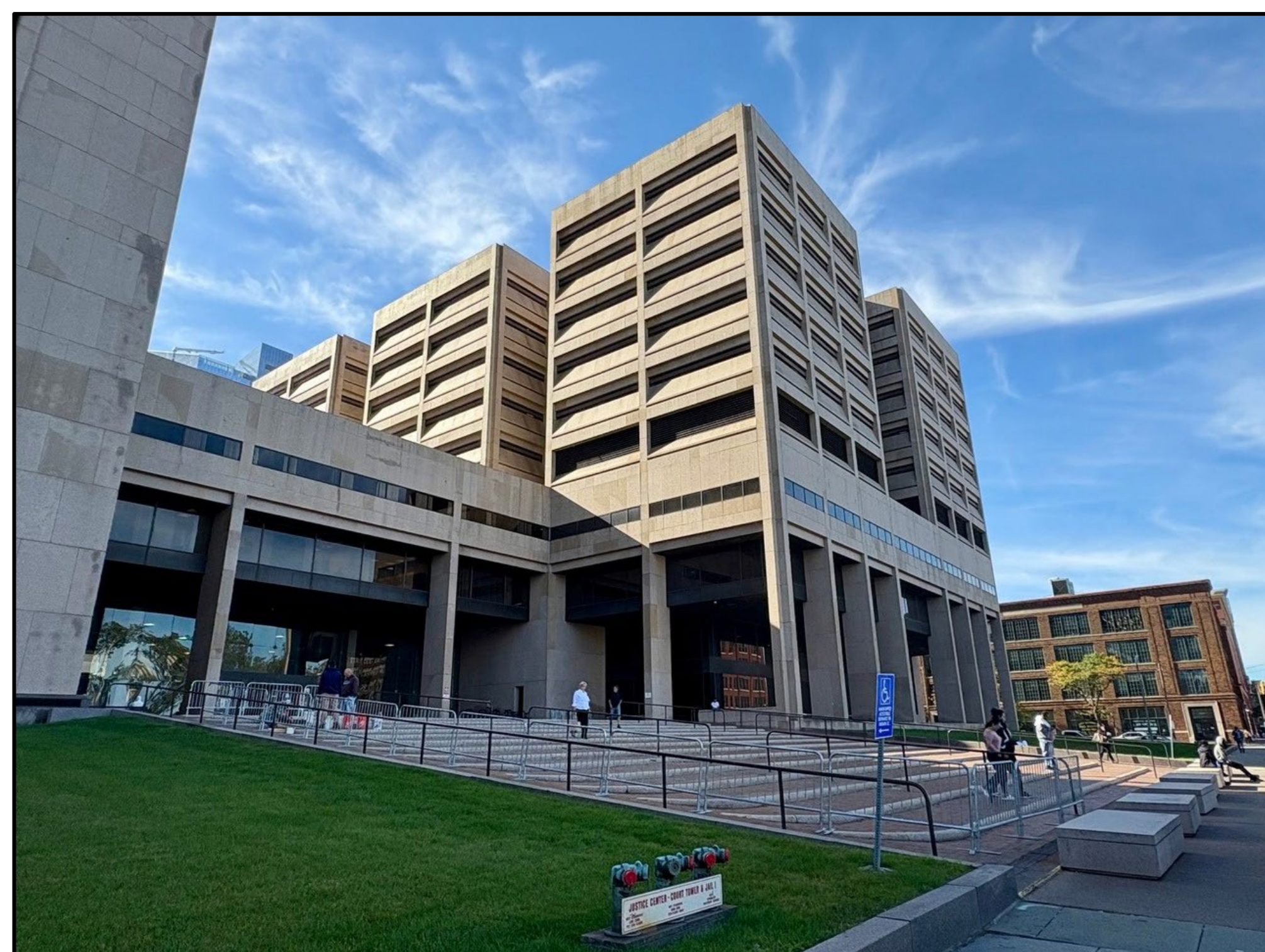
Figure 1: Cuyahoga County Corrections Center (CCCC) located within the justice center complex in downtown Cleveland
