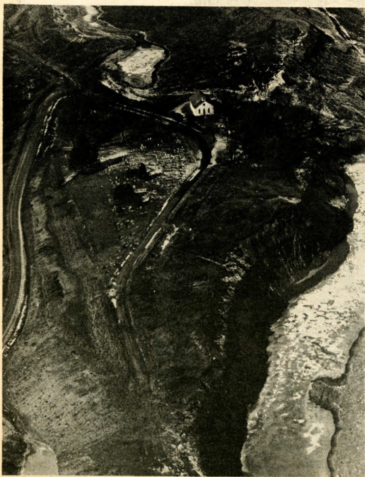
Salem Church outside the town of Egypt, Ohio in Belmont County. Hanna Coal Co. stripped this area, completely destroying the town of Egypt. Salem Church is all that is left of the town. Hanna Coal had the abandoned Church painted white.
